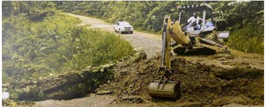
Machine mobilised for repair
