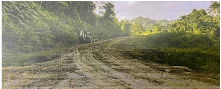
Repair work completed
